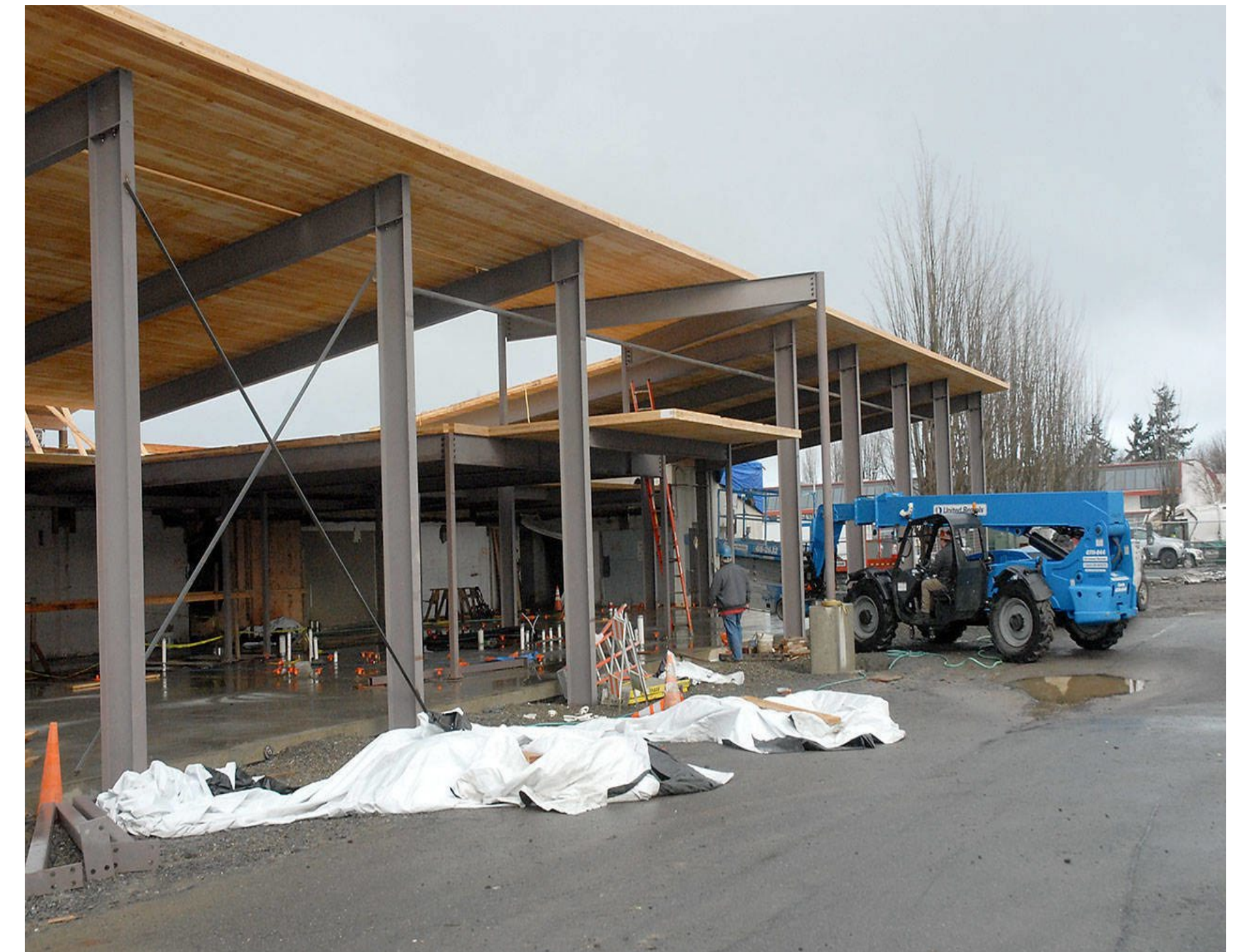
CLT for roof at Shore Aquatic Center
